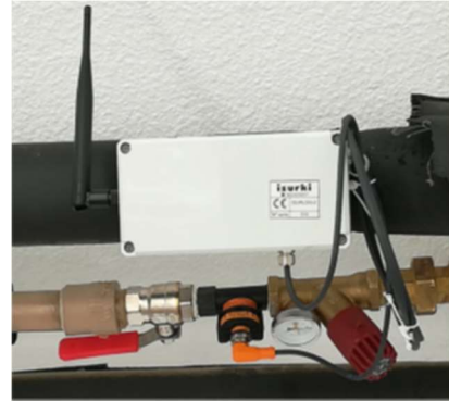
ISURLOG Compact deployed unit remotely monitoring flow and temperature on a hot water distribution network with LoRa comms.
